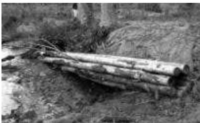
Newaukum 2 project is on a small fork of the main stream. The installed structures have a length that is more than twice the bank-full width, and a diameter more than three times the typical flow depth. Although the structures appear oversized for the location (given current notions of habitat enhancement), they are of the size and scale of trees native to the area. The project was installed during early 2000, so long-term performance is yet to be assessed.
