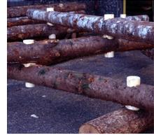
Spars provide an all-wood structural connector between crossing poles. The hole bored through each pole is tapered so that a solid mortise and tenon joint is created as a wedge is driven into each end of a connecting spar. Round wooden mortise and tenon joints enable the structure to flex and adjust to hydraulic loads as well as changes in streambed form.
