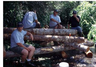
The fall rain season has produced rainfall at least fifty percent above normal, and a number of rain-on-snow events. To-date the engineered log jams have performed exactly as expected. Flow through the structures is as anticipated. Scour and deposition of gravel is dramatically improving what was previously a plane bed channel. Fine organic debris is accumulating on the structures, thus delaying its movement through the system.
